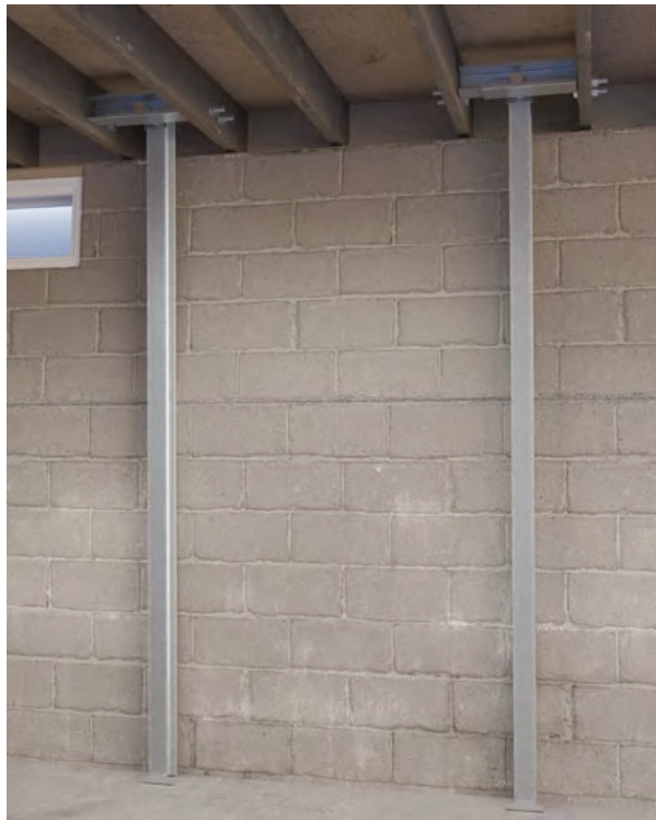
Figure 3.25 PowerBrace installation with joists perpendicular to wall
